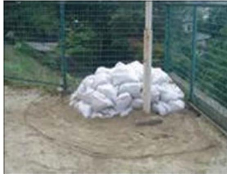
Figure 13: Temporary storage of contaminated material – examples from clean-up demonstration tests
