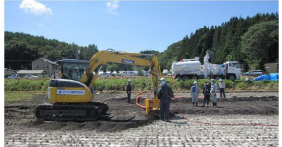
Figure 3: Testing top soil removal after using soil hardener (Courtesy of MAFF-JAEA-NARO).
