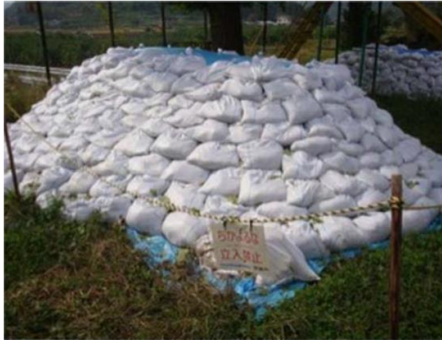
Figure 13: Temporary storage of contaminated material – examples from clean-up demonstration tests
